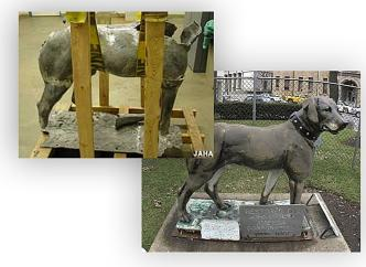
The repairs involved a process known as lead-burning, a technique similar to soldering. The dog was filled with concrete and reinforced with steel rods, then coated with fiberglass "skin" to protect him from the weather. Morley's dog returned to his place in the park before Kline's Store in November of 1973.
